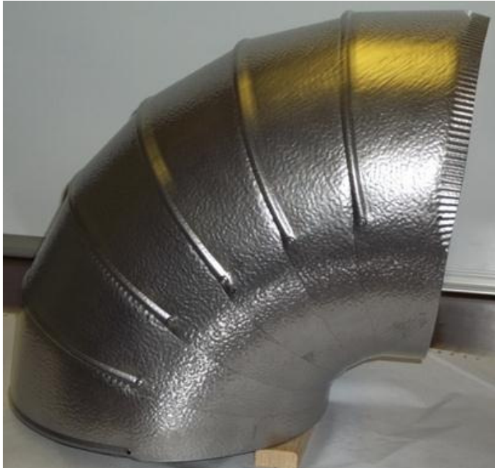
Figure 11 – Finished mitered metal jacket sections (gores) applied to elbow over mass loaded vinyl.
