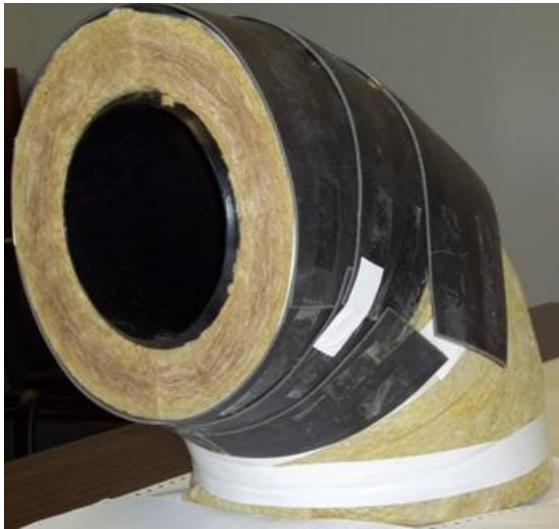
Figure 7 – Mass loaded vinyl mitered sections (gores) placed around insulation with longitudinal joint at about 3 o'clock and with required \geq 1.3 cm ( \geq \frac{1}{2} inch) longitudinal overlap. Also shown is overlap at circumferential joint which is required to be a maximum of 1.3 cm ( \frac{1}{2} inch).
