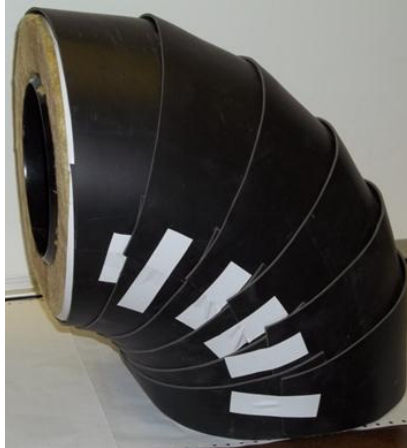
Figure 8 – Tape or staples are used to lightly secure mass loaded vinyl mitered sections (gores) in place at both longitudinal and circumferential joints.
